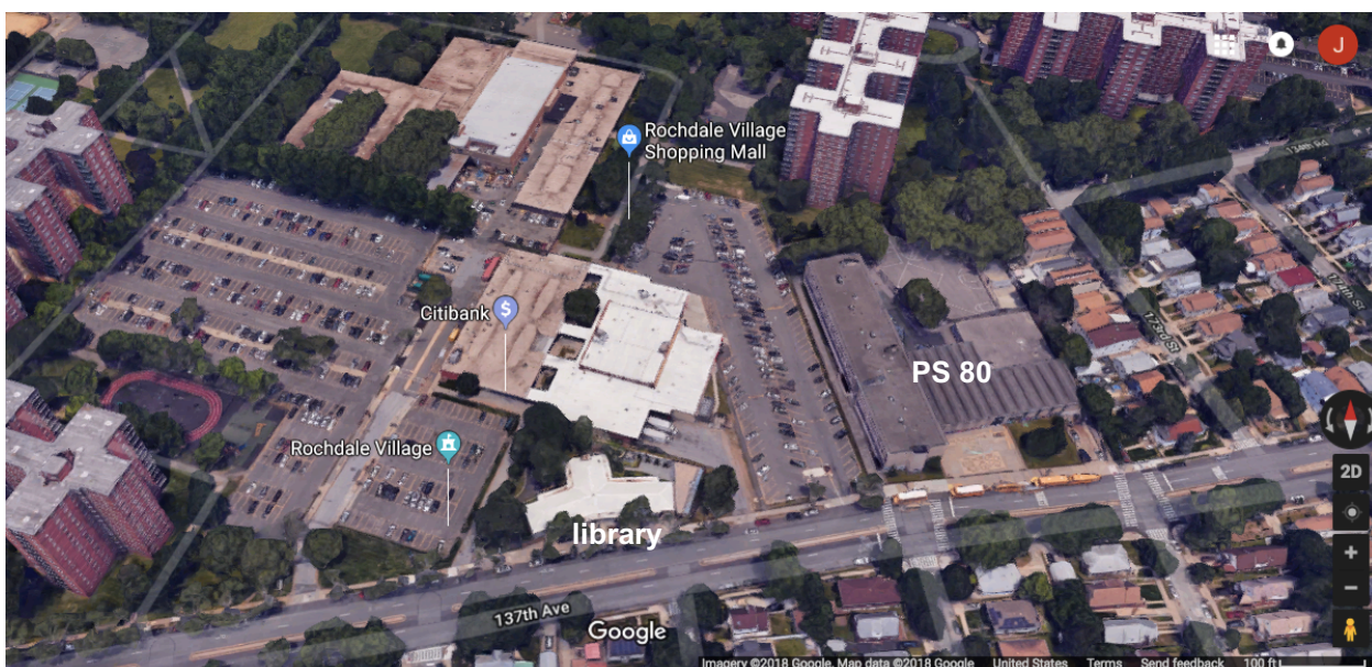
Zoom in to Rochdale Village Shopping Mall #2; adjacent uses are PS 80 Thurgood Marshall Magnet School and Queens Library at Rochdale Village. https://www.rochdalevillage.com/mall2/listing
