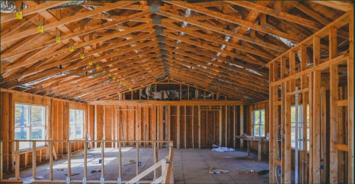
Shell House Programming Center (unfinished), Roots to Sky Sanctuary Site, Oakland, MD
