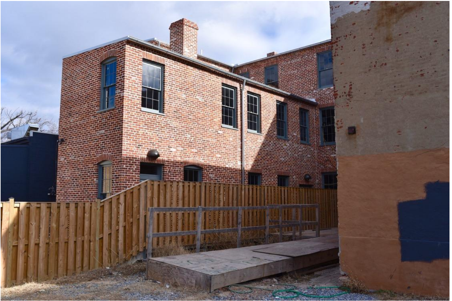
Figure 25. View of Woodson home looking northeast, showing south elevation of rear ell, January 2018. NPS Photo. (DC_Washington_Carter G Woodson Home_0005)
