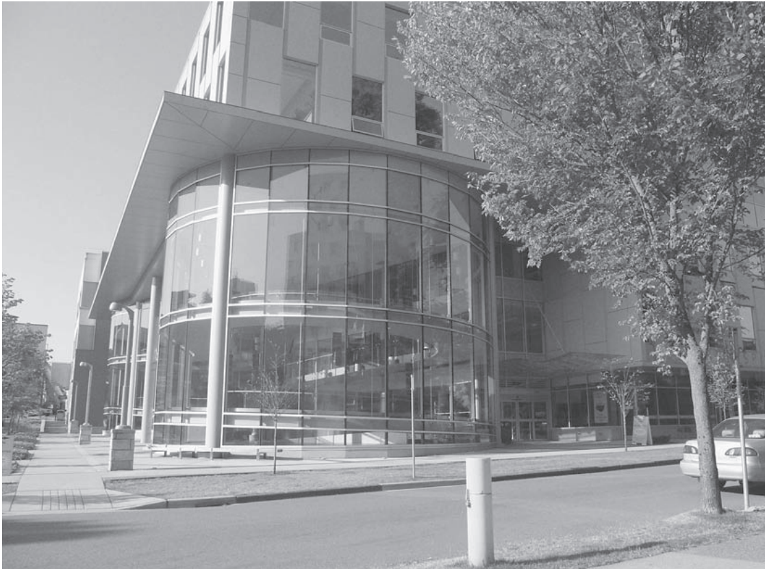
Figure P.1. The glass and steel structure of the Blusson Spinal Cord Center in Vancouver, British Columbia, discloses a glass atrium with a winding, colorful ramp (2010). Photograph by author.
