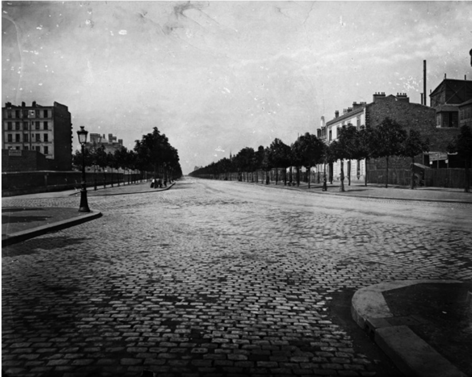
FIGURE 14. Charles Marville, photograph of Boulevard Arago, Paris, date unknown but possibly 1865–68. The photograph shows a large, empty, paved intersection of boulevards in Paris. The street has a pronounced curved profile. To the right and left are raised sidewalks with high curbs. Rows of planted trees line the space between the pedestrian area of the sidewalks and the street.
