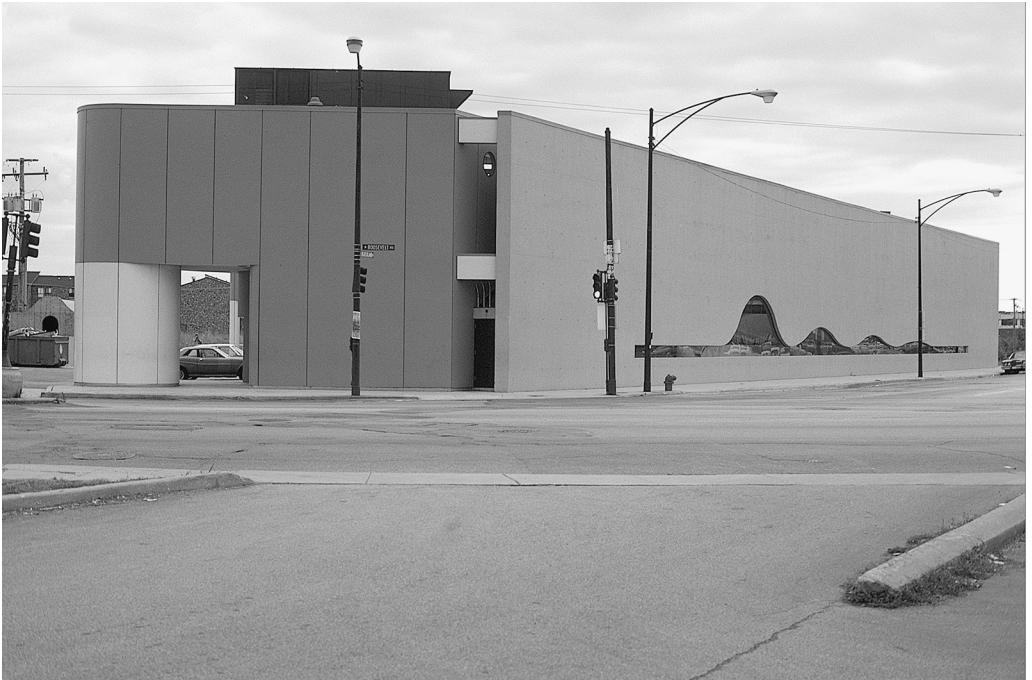
Figure 5. Northern and western exposures of Illinois Regional Library for the Blind and Physical Handicapped, ca. 1978, from the corner of Roosevelt Road and Blue Island Avenue. Note car-shaped garage under construction, behind dumpster, in left background. Copyright Massachusetts Institute of Technology. Reproduced from the G. E. Kidder Image Collection at the Massachusetts Institute of Technology under a Creative Commons Attribution-Non Commercial 3.0 License.
