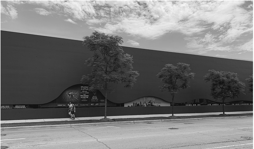
Figure 7. Western wall facing Blue Island Avenue set with waveform window, now used to advertise bank services. Photograph taken July 2019 by Brian Selznick.
