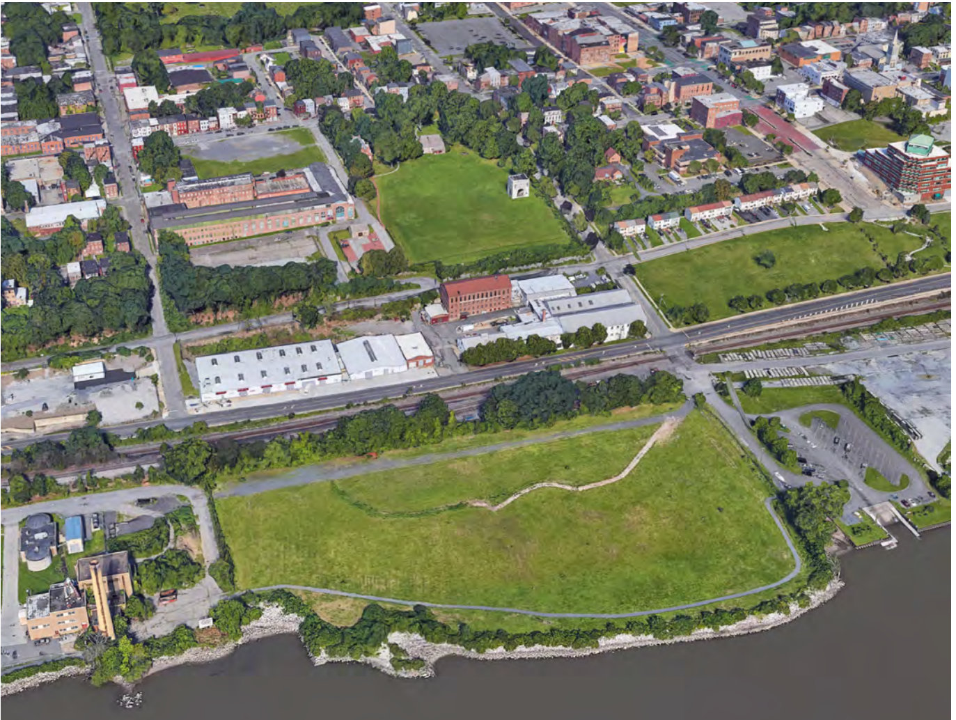
Aerial of Newburgh
