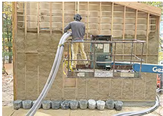
Left: Straw panel construction using EcoCocoon prefabricated panels, right: Spraying hemp lime at Wally Farms
