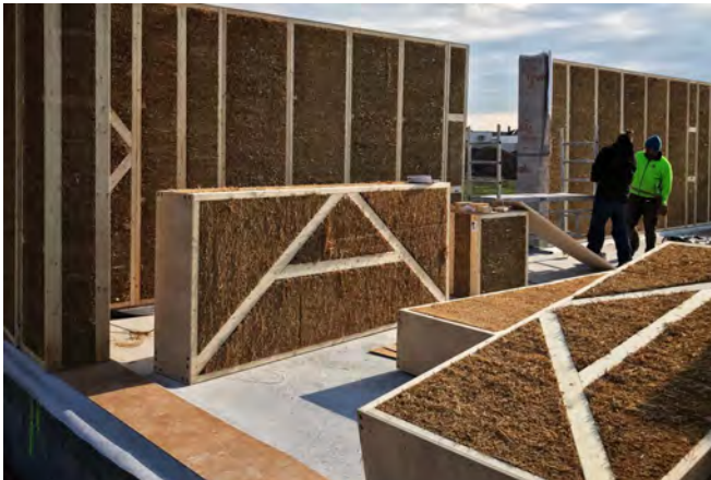
Left: Straw panel construction using EcoCocoon prefabricated panels, right: Spraying hemp lime at Wally Farms
