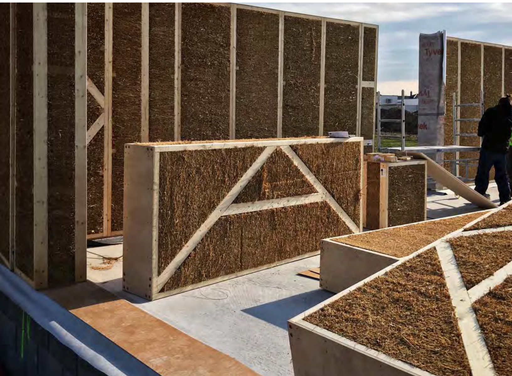
Ecococon panels on site for install
