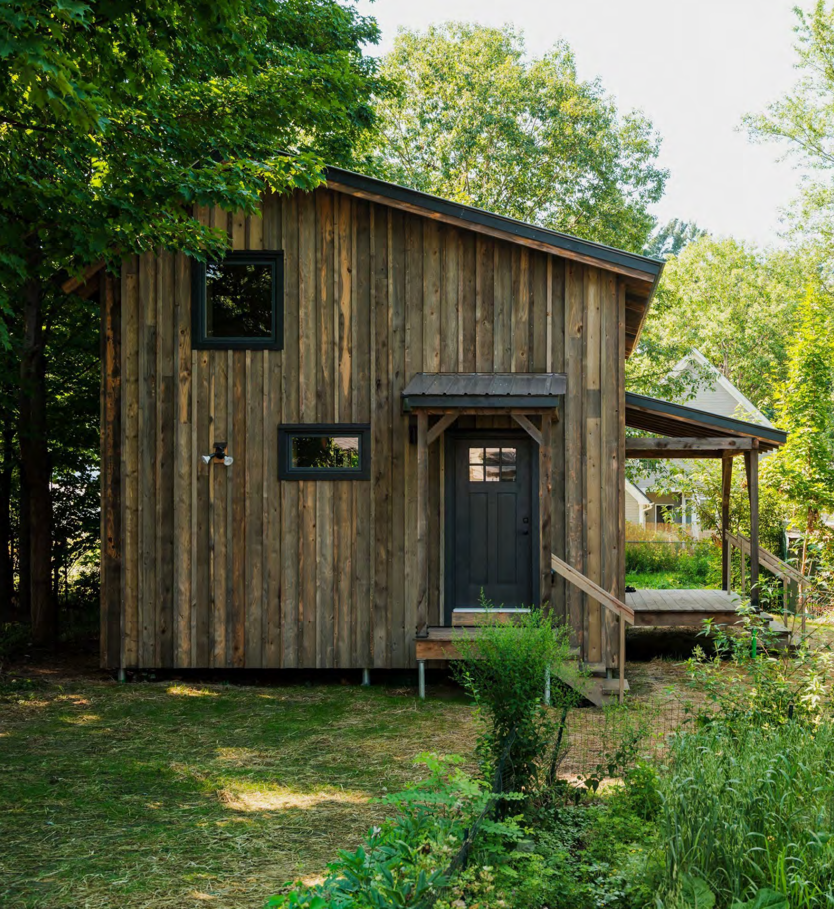
Image: Terra 600, Burlington, VT designed and built by New Frameworks is a 600 sf ADU in the backyard of a single family home. Straw panels were prefabricated at New Frameworks' facility and then transported and installed. Image Credit: New Frameworks
